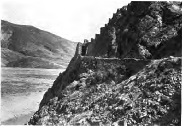
FORTIFIED WALL ACROSS THE ROAD NEAR PIN-DZO-LING.
